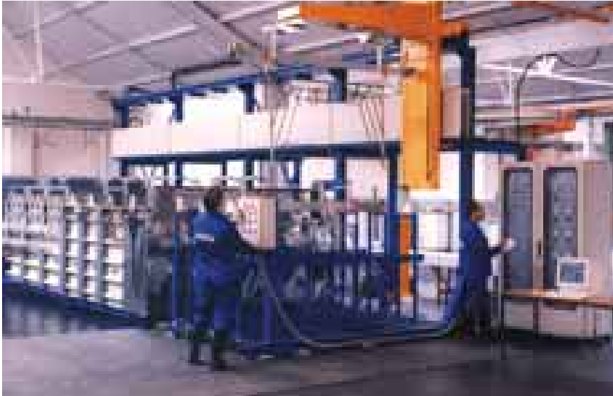
Photo provided courtesy of Anopol Ltd
