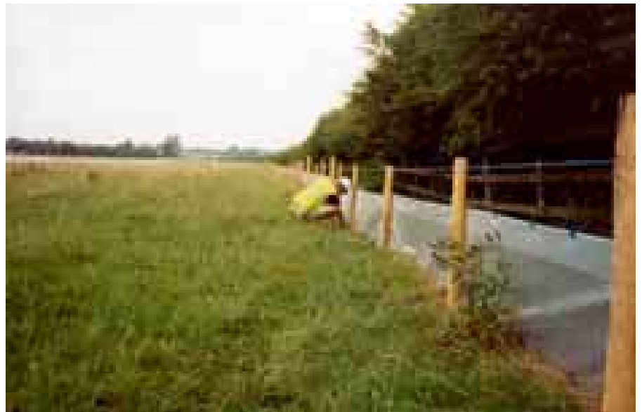
Example of amphibian fencing used to exclude great crested newts from a development area.
